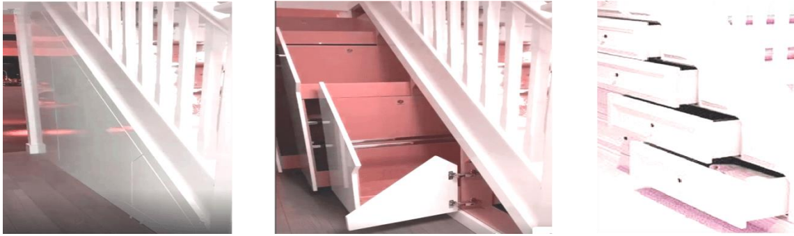
Fig. 2 Storage drawers under the stair (created by the authors)
