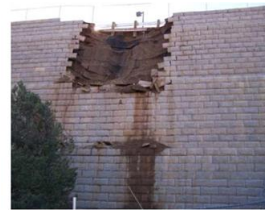
(d) Built in 2016, movement occurred after being measured with an inclinometer 2021 location Fort Mill Township York County South Carolina, USA
